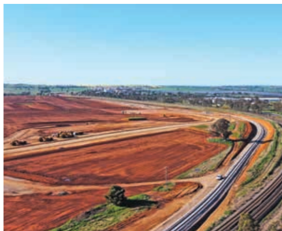
Riverina Intermodal Freight and Logistics Hub, New South Wales
