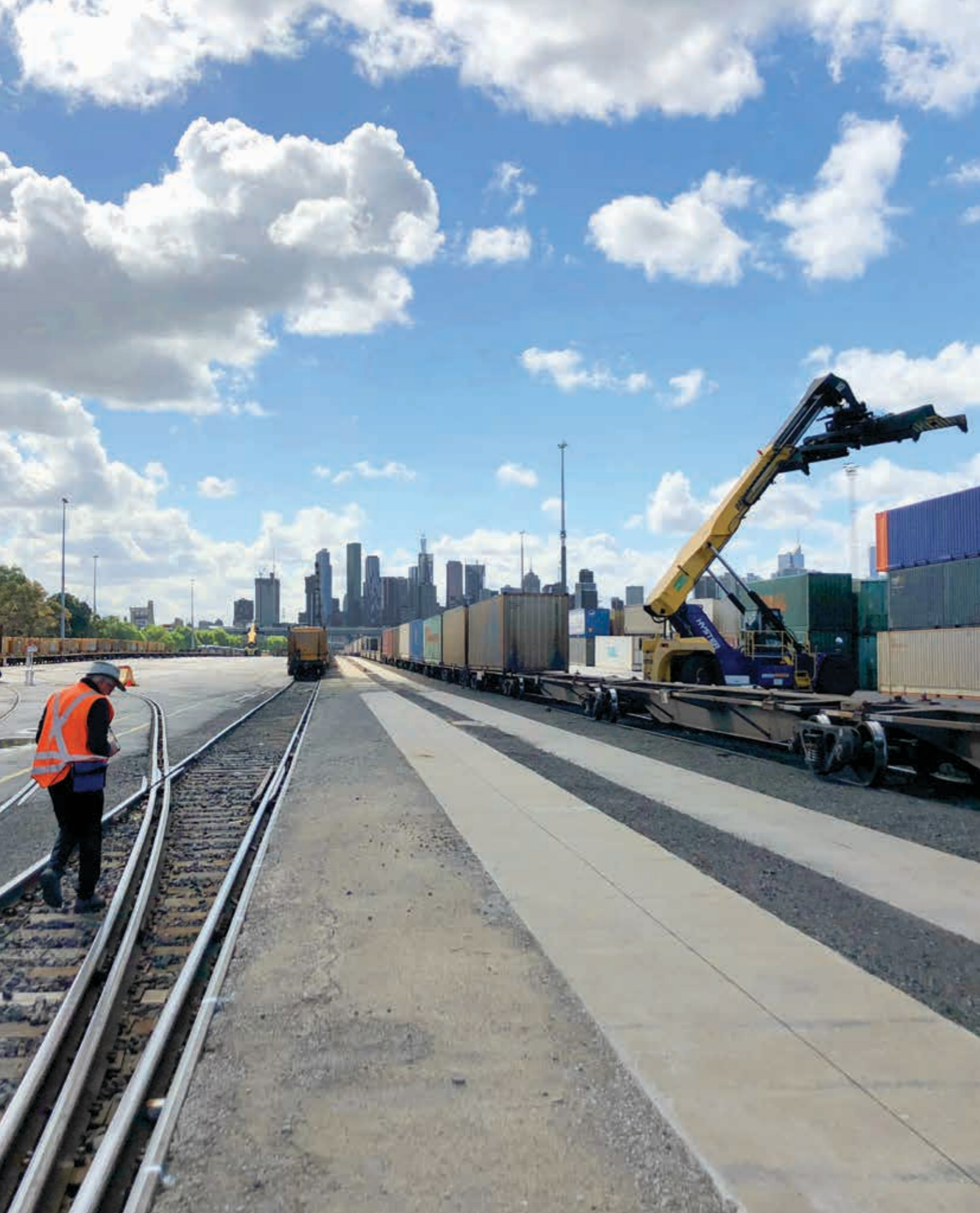
Track inspection, Melbourne, Victoria
